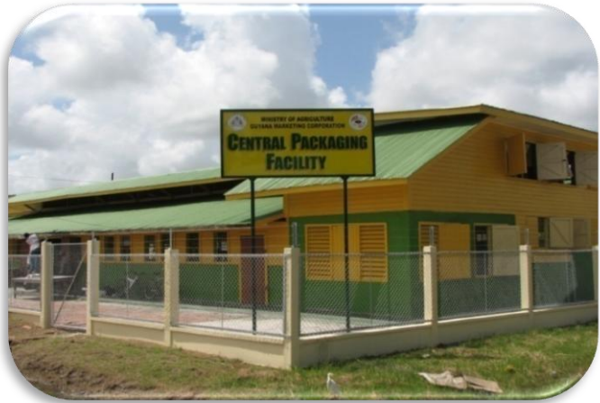
Figure 27: Central Packaging Facility (CPF)
